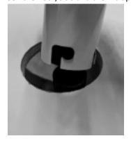
7. Slide the Drain Kit on the ABS or PVC 1 ½" pipe making sure it sits flat on the floor. \*
