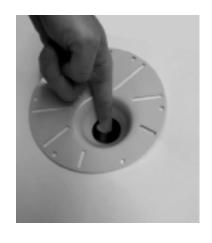
12. Apply provided lubricant inside the Drain kit. Please only proceed with this step once the pressure test has been performed, if needed.
