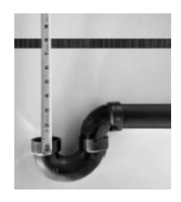
3. Measure the distance from the inside of the P-trap to the top of the floor or slab. (P-Trap not included)
