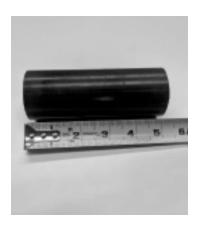
4. Cut the ABS or PVC 1 ½" pipe 3 inches shorter than the distance between the floor/slab and the P-trap.
