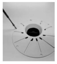
9. Secure the Drain Kit to the subfloor/concrete with screws or cement.
