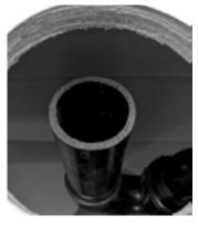
5. Apply glue to the outside of the ABS or PVC 1 ½" pipe and to the inside of the Ptrap. Insert the pipe into the P-trap.
