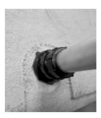
13. Affix the appropriate tailpiece to the waste & overflow. Ensure the measurement between the base of the Drain kit and the P-trap will accommodate the tailpiece.
